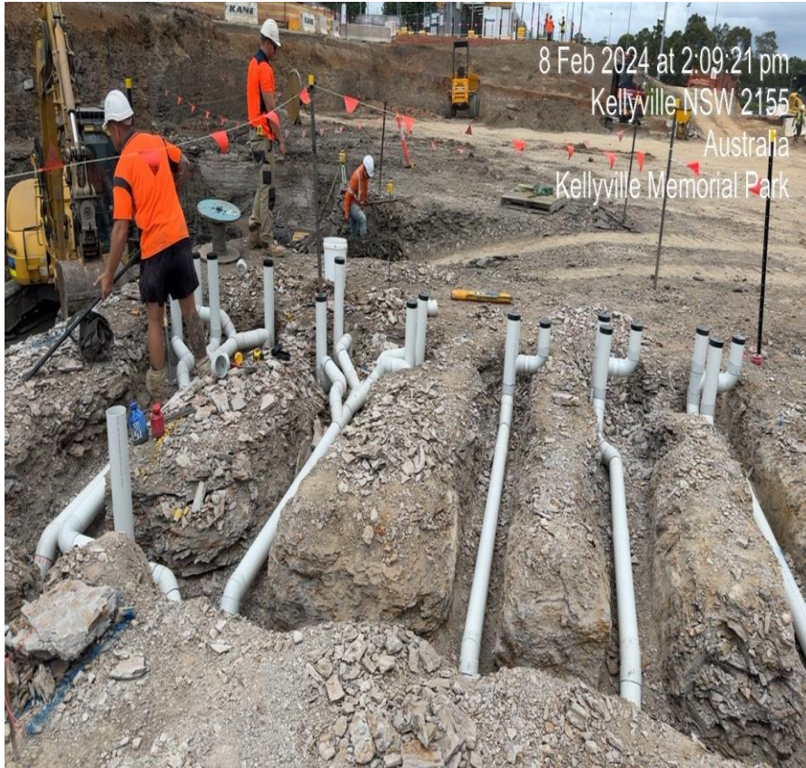
Building B – Inground drainage works
