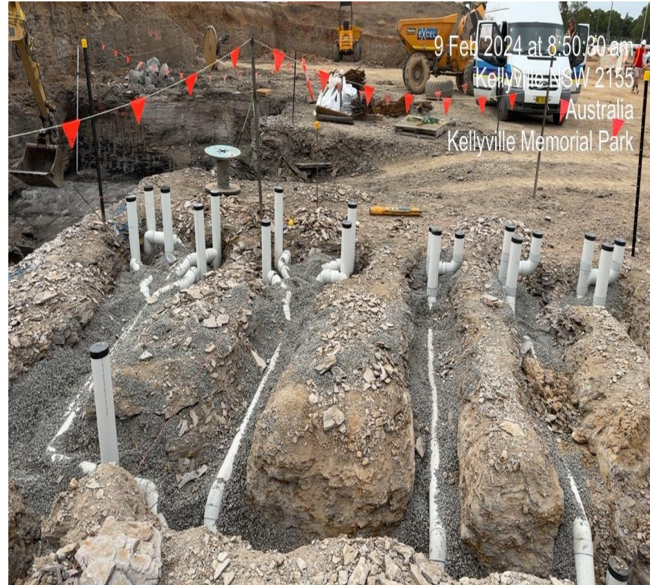
Building B – Inground drainage works
