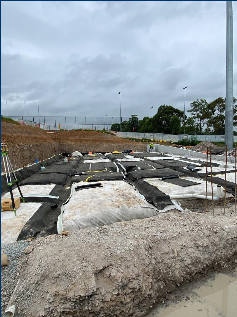
Building A – MastaTex Installation
