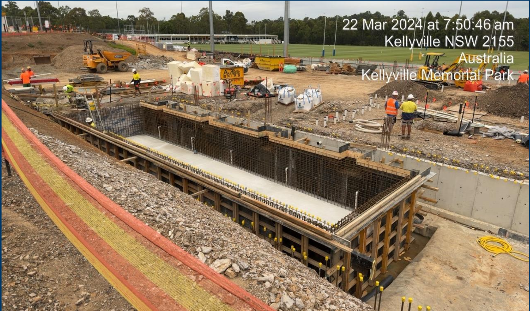
Pool base complete
