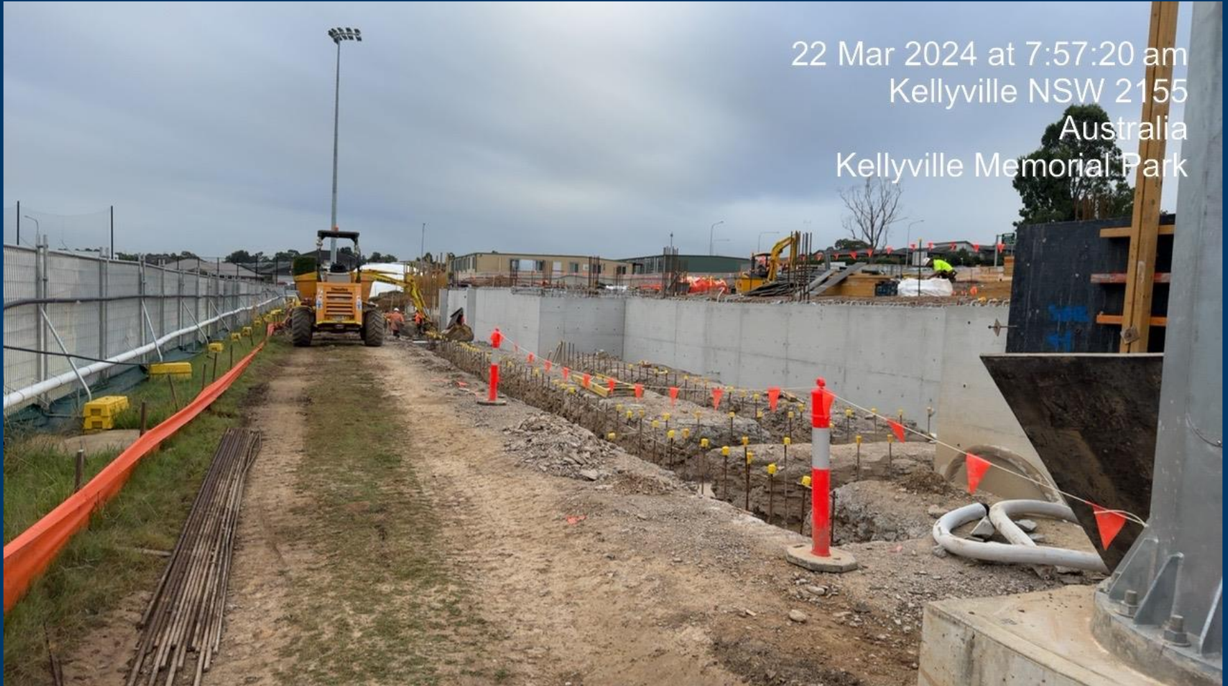
Building B- Walls
