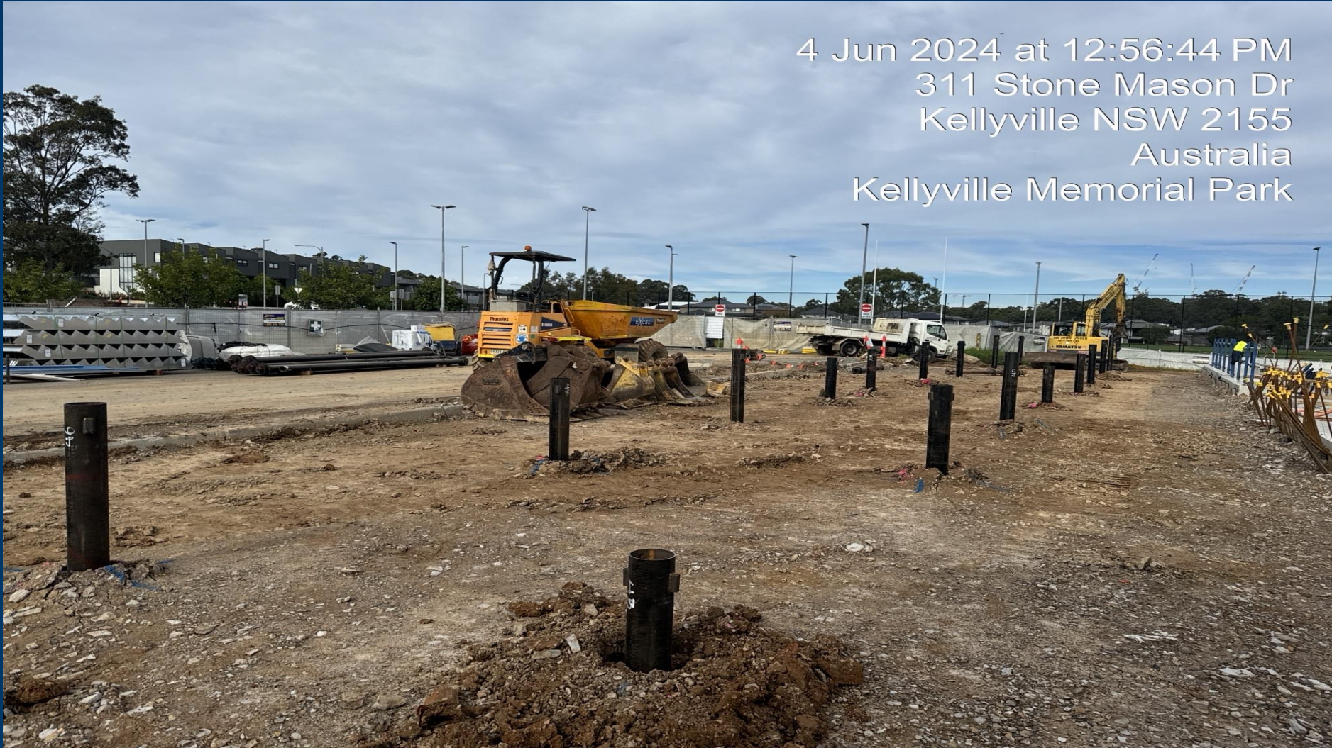
Building A – Screw Piling
