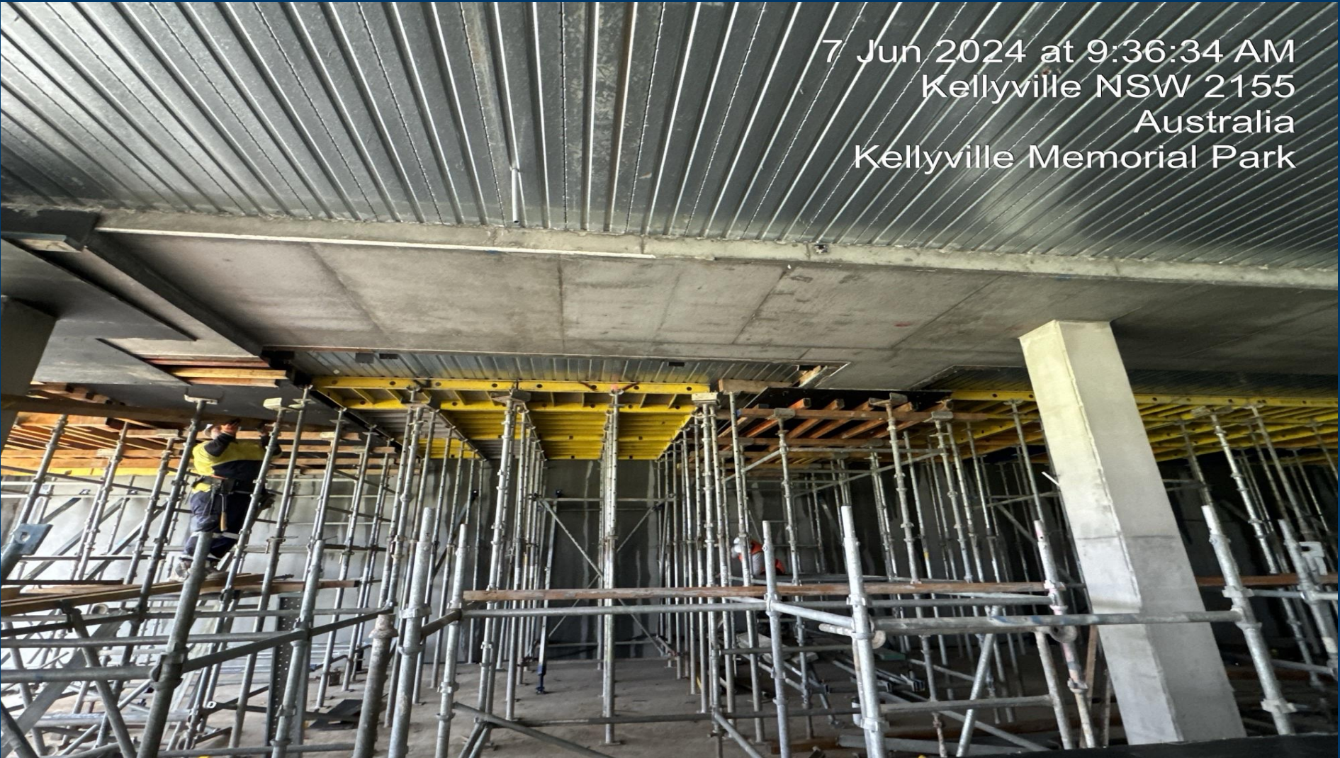
Building B – Formwork Stripping Suspended Deck Pour 1
