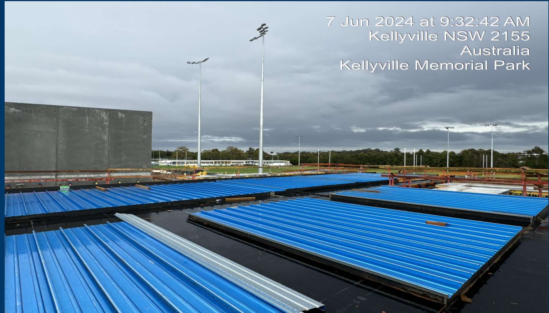
Building B – Bondeck to Suspended deck Pour 2
