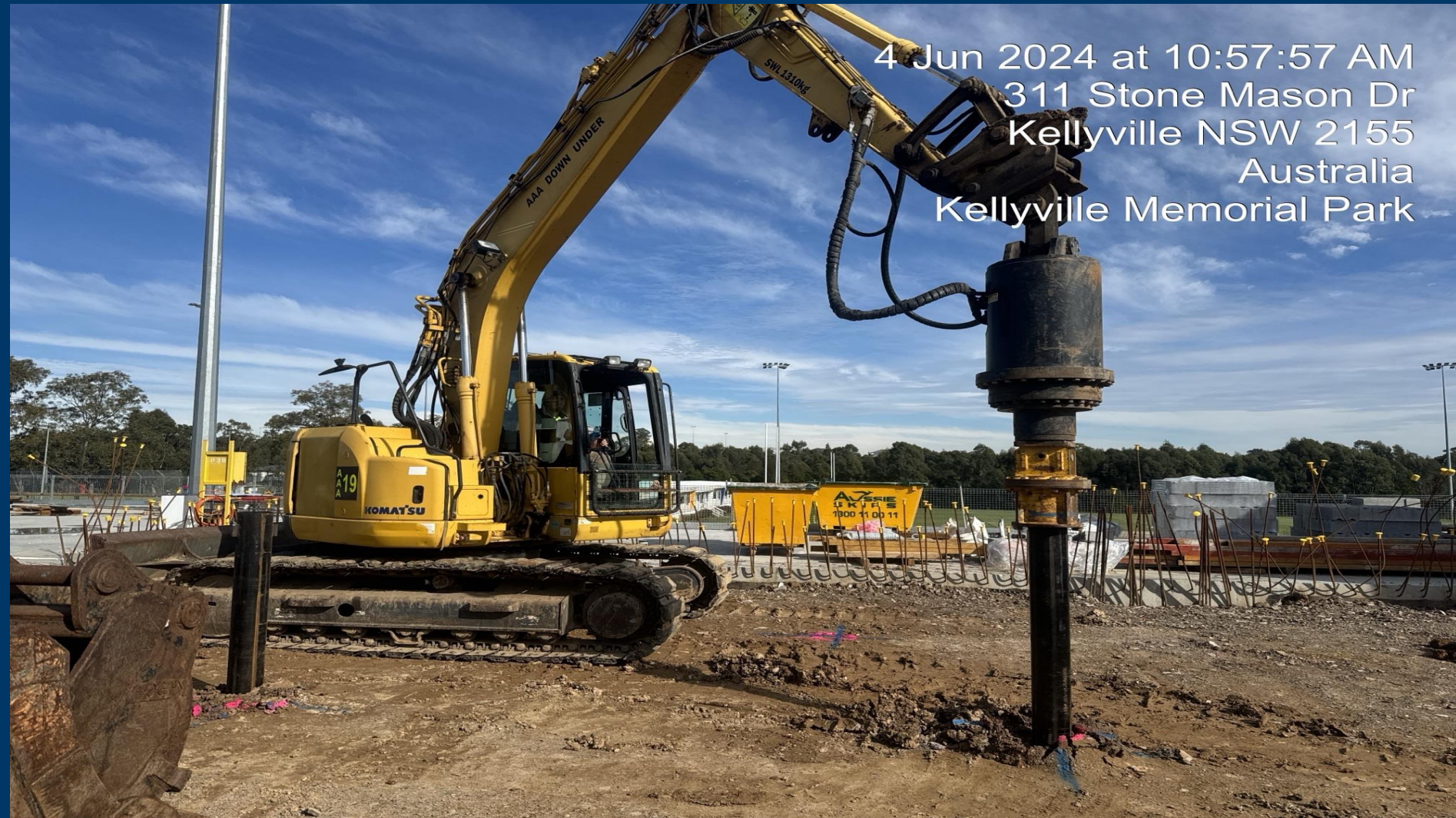
Building A – Screw Piling Installation
