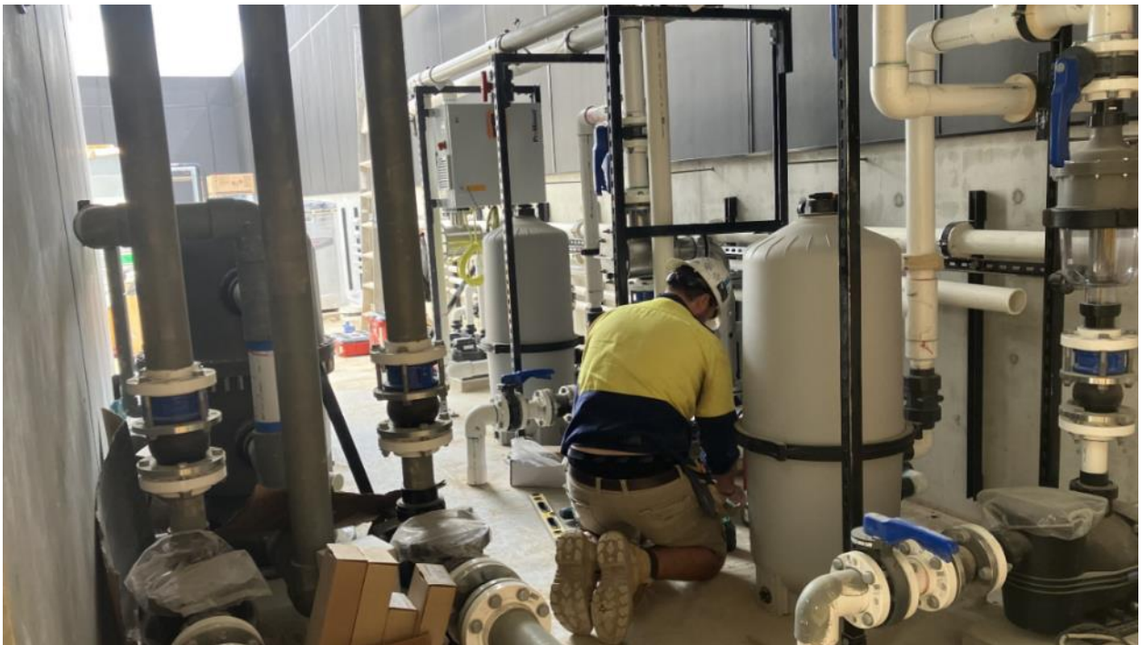
Indoor pool filtration system
