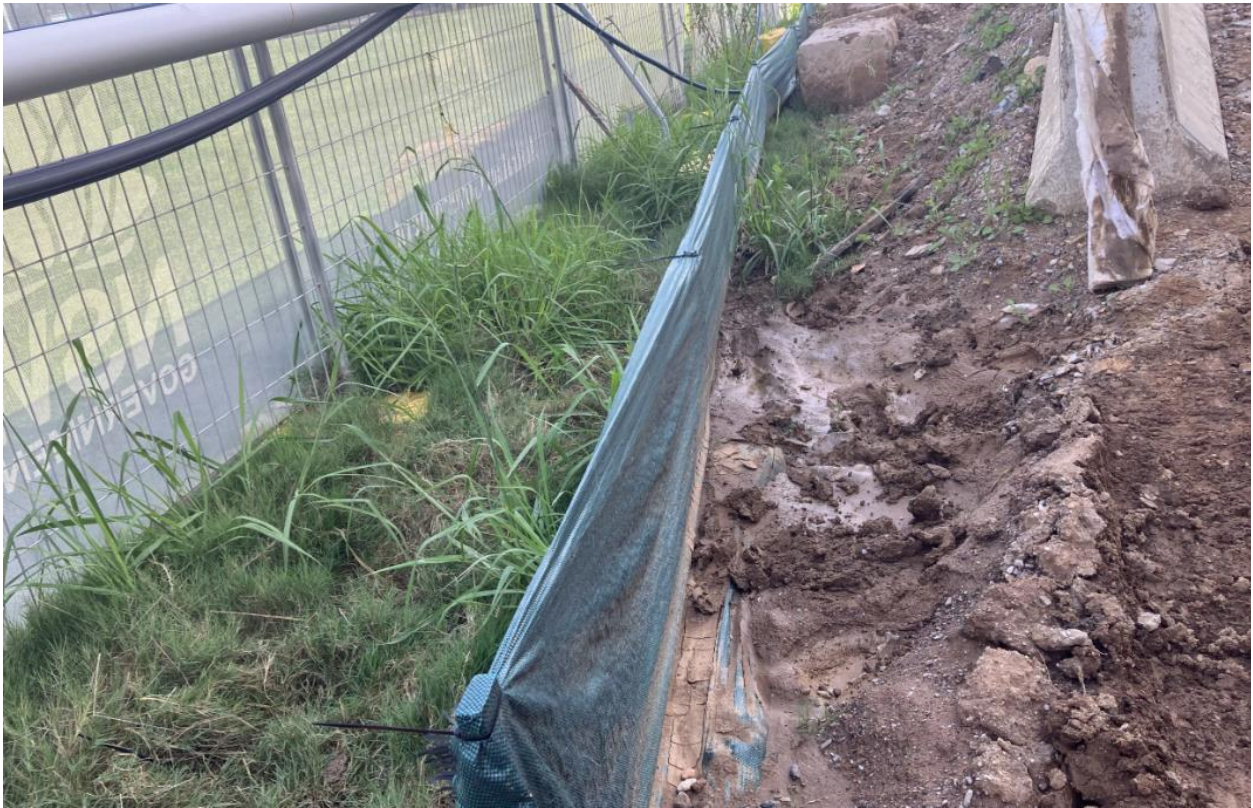
Sediment fencing at boundary fence
