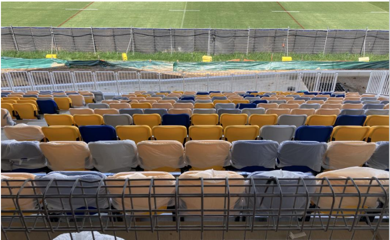
Seats, fencing and guardrails installed. Seeding to occur at boundary; once established, sediment fencing will be removed.
