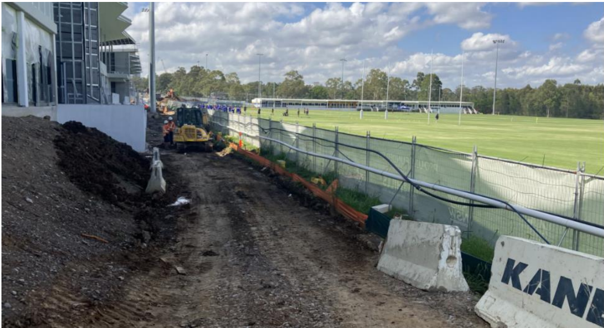
Batter being topsoiled in preparation for landscaping works
