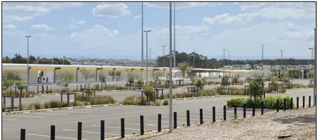
Figure 9 | View of the CF from existing carpark (source: Applicant)
