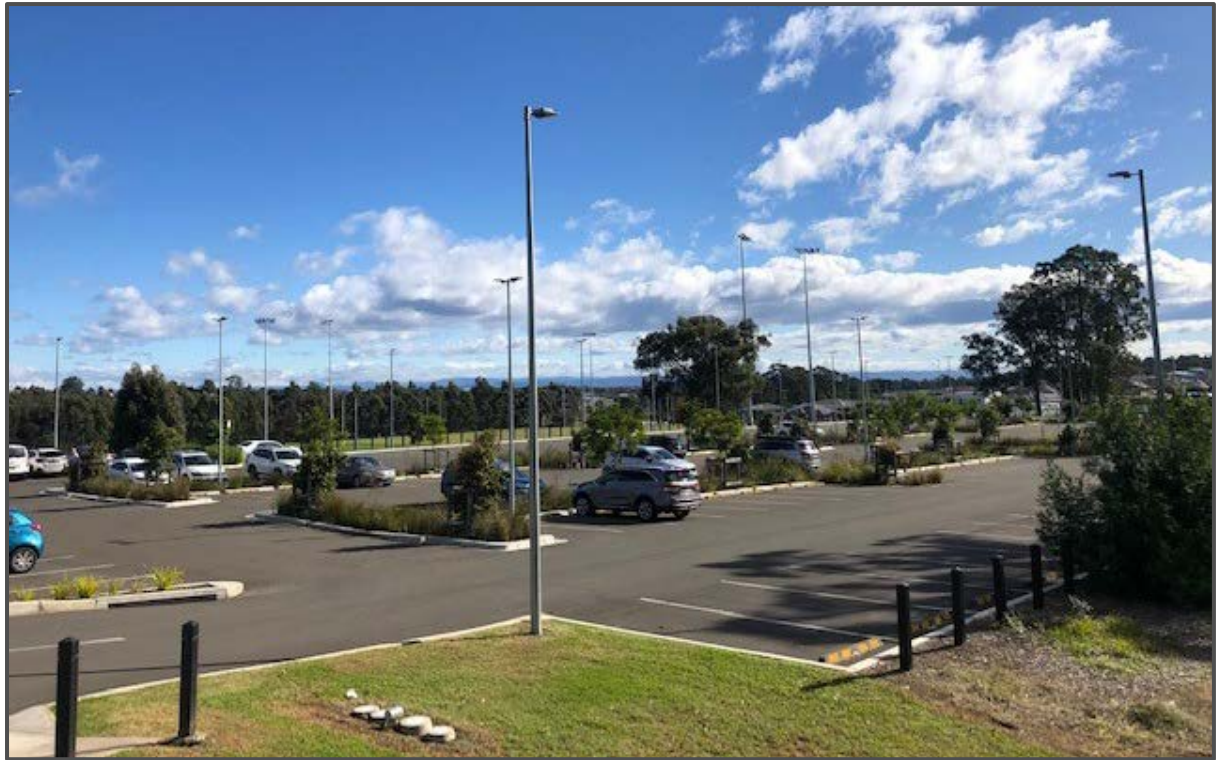
Figure 3 | Existing at-grade carpark with 223 spaces accessed via Stone Mason Drive looking north-west (source: Department)
