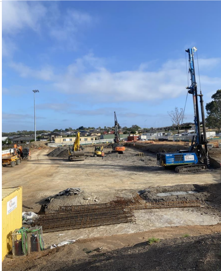
Piling has been completed
