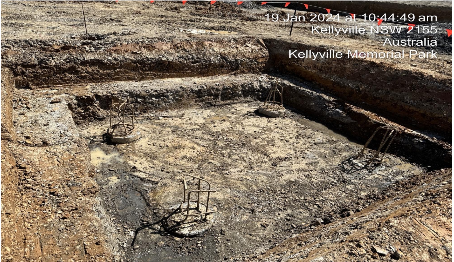
Lift pits ready for waterproofing Building B
