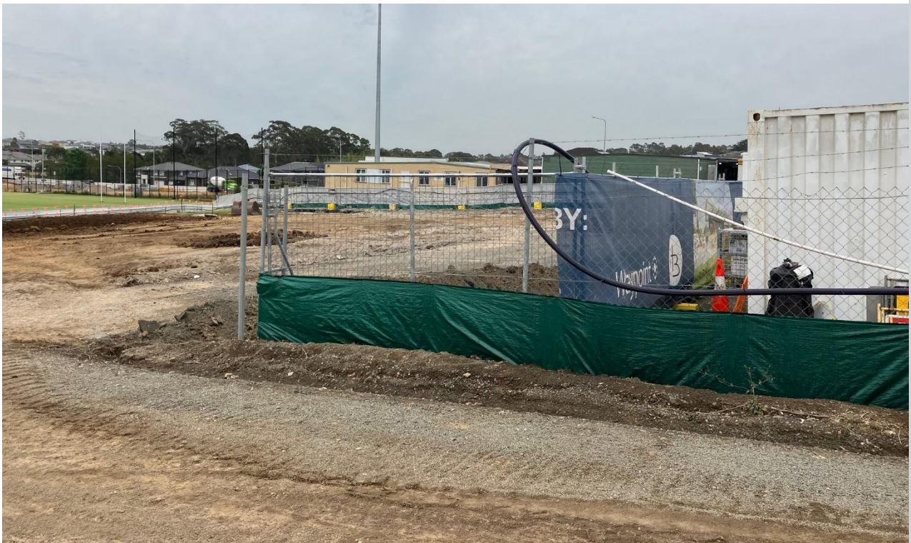
Sediment fencing installed at border with Daracon site.
