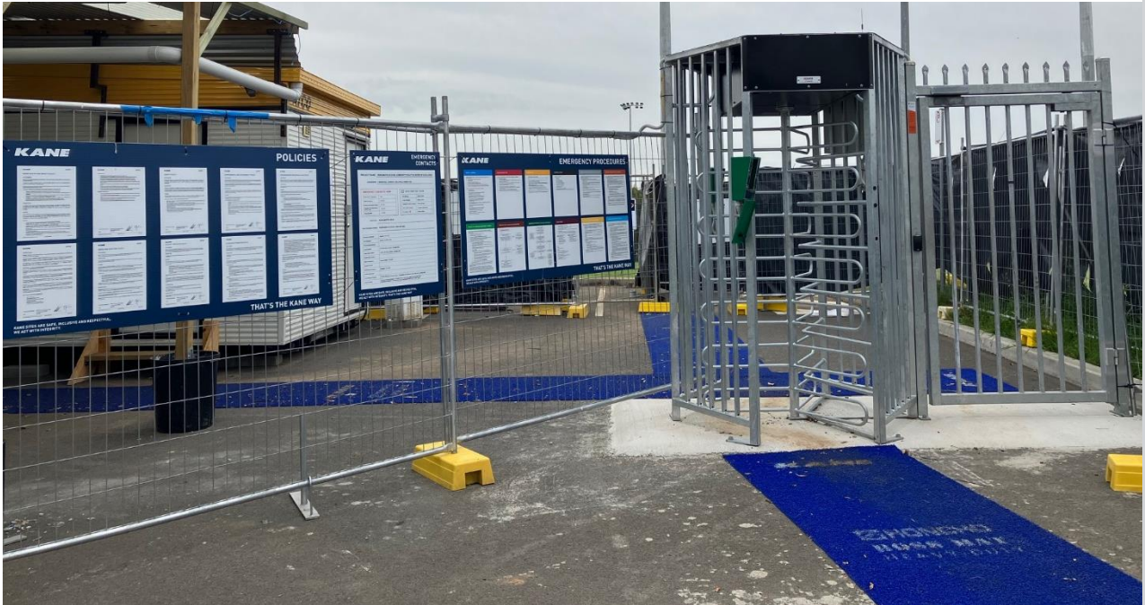
Project information on display and secured turnstile to Site. Site accessible using face recognition application. Designated blue walkway throughout the site.
