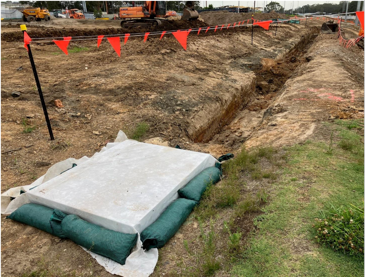
Protection of pit drain. Sediment basin being excavated. Work has stopped in this area due to unexpected find. Pipe to be sampled by hygenist and sent for testing.
