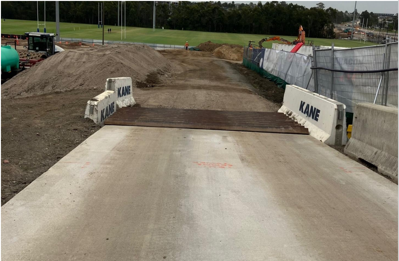
Rumble grid and hardstand at site access/egress.
