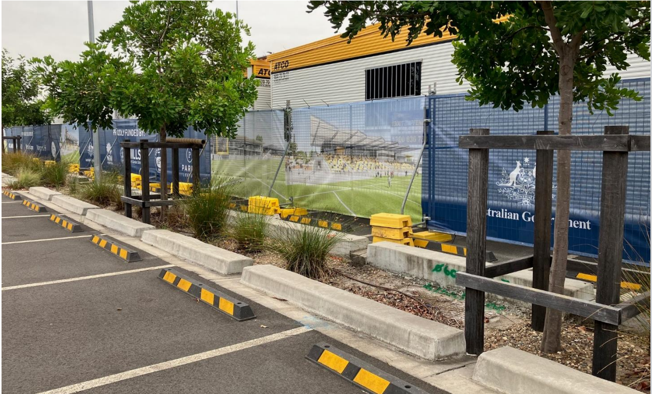
Fencing with shade cloth installed at existing carpark.
