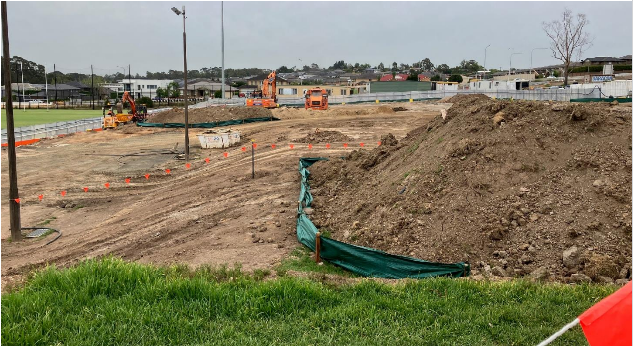
Excavated material topsoiled for reuse onsite. Sediment fencing installed.
