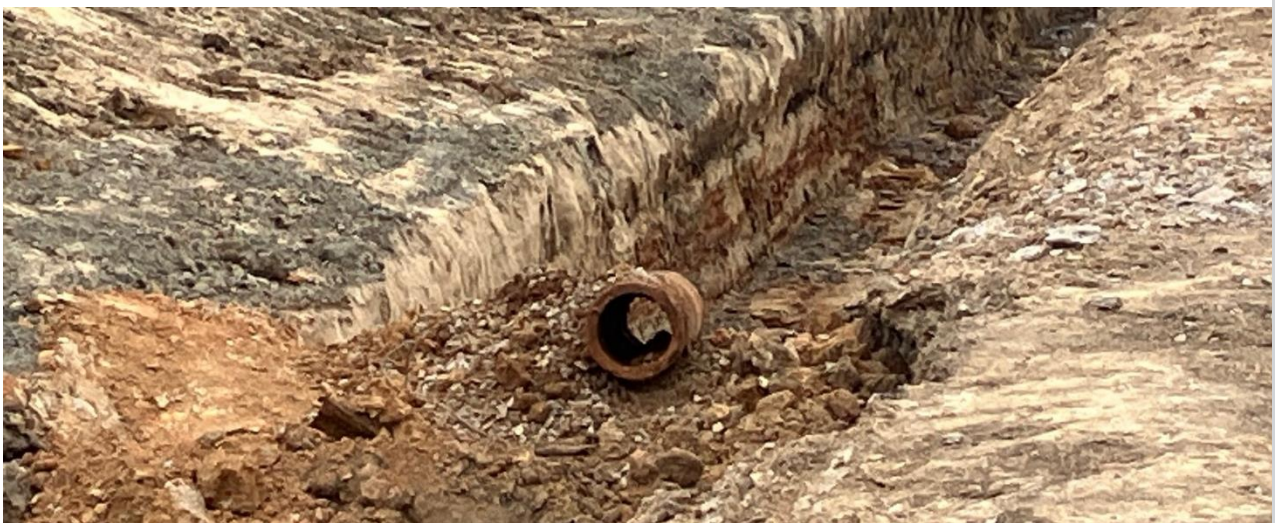
Protection of pit drain. Sediment basin being excavated. Work has stopped in this area due to unexpected find. Pipe to be sampled by hygenist and sent for testing.
