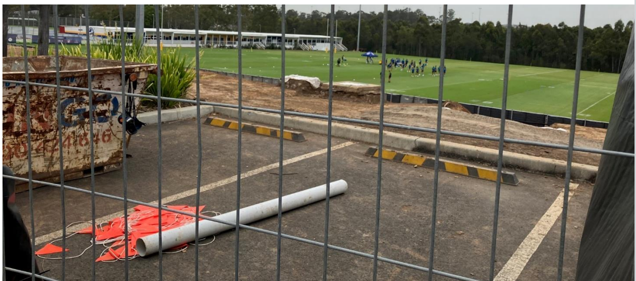
Previous location where asbestos was stored, now removed.
