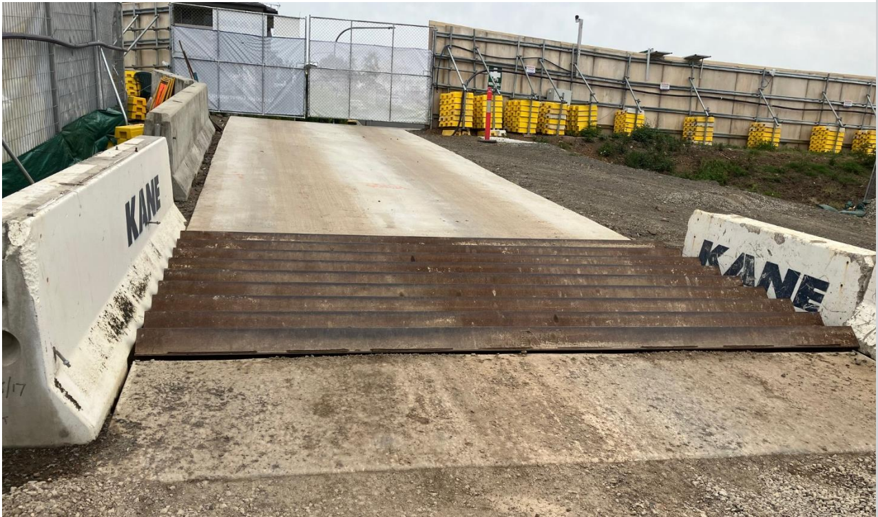
Rumble grid and hardstand at site access/egress.
