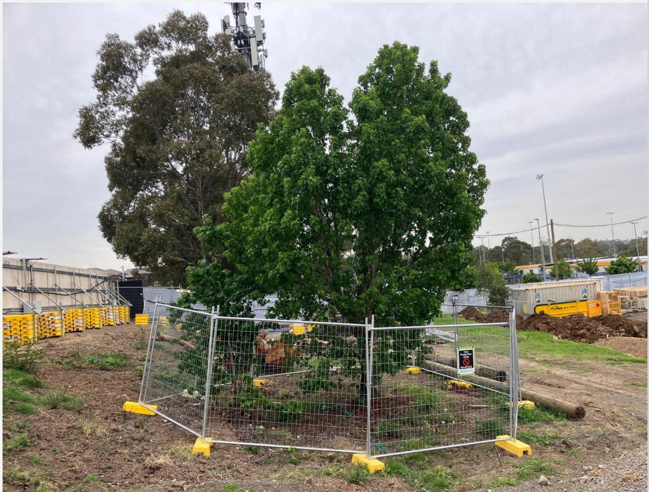
Tree protection in place.
