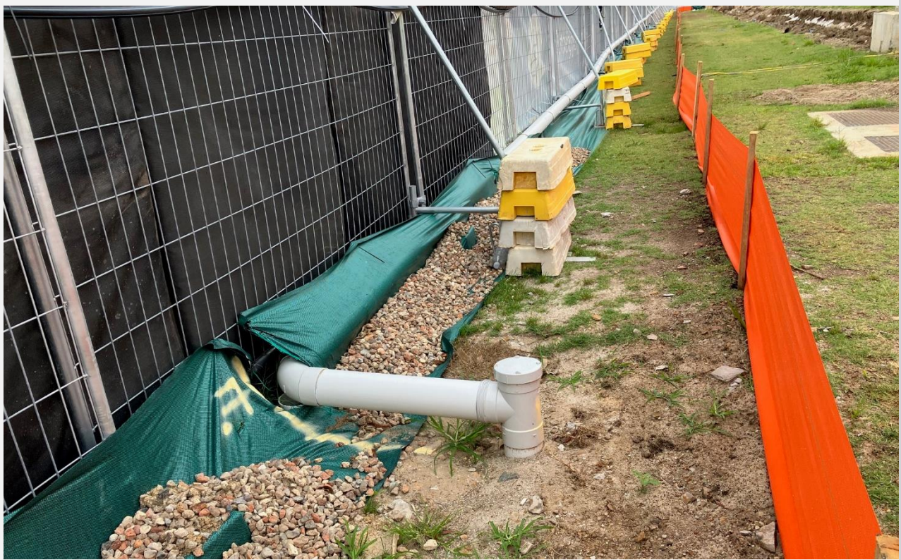
Potable water connected to service the site. Sediment fences installed along the perimeter.
