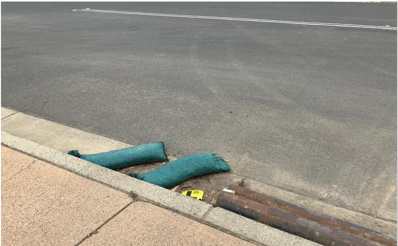
Sandbags in place at site exit.
