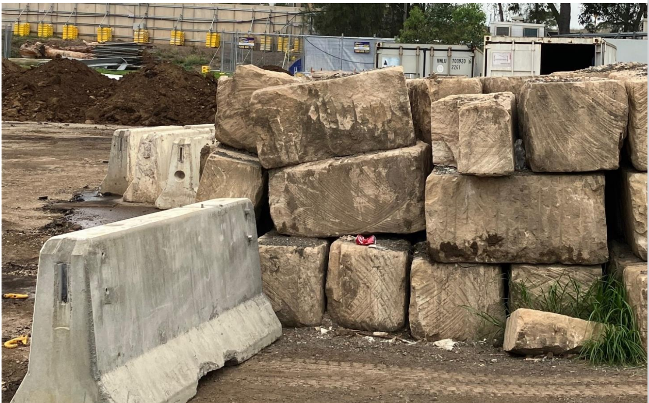
Excavated sandstone with plans to incorporate into the development.
