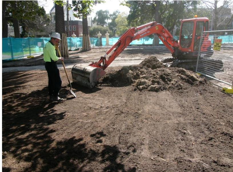
**Figure 1** – Showing method for removal of residual surface vegetation from Tree Protection Zones following herbicide treatment and slashing.
