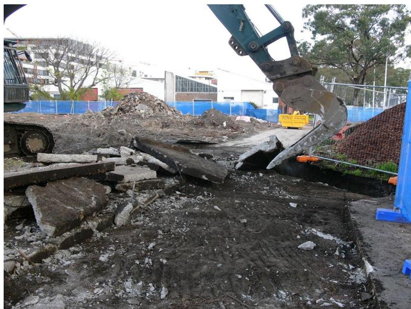
**Figure 2** – Showing method for removal of concrete pavement, by carefully lifting sections and folding over the remaining paved surface.
