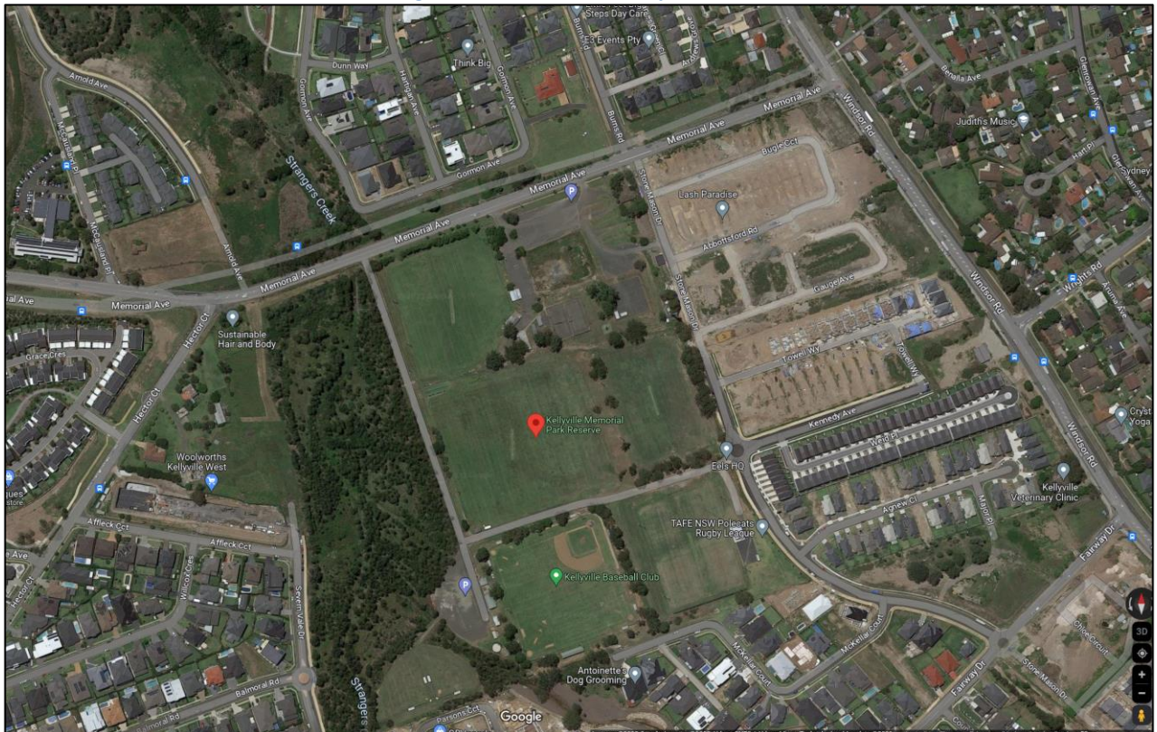
Figure 2 : Aerial View of the Subject Site
